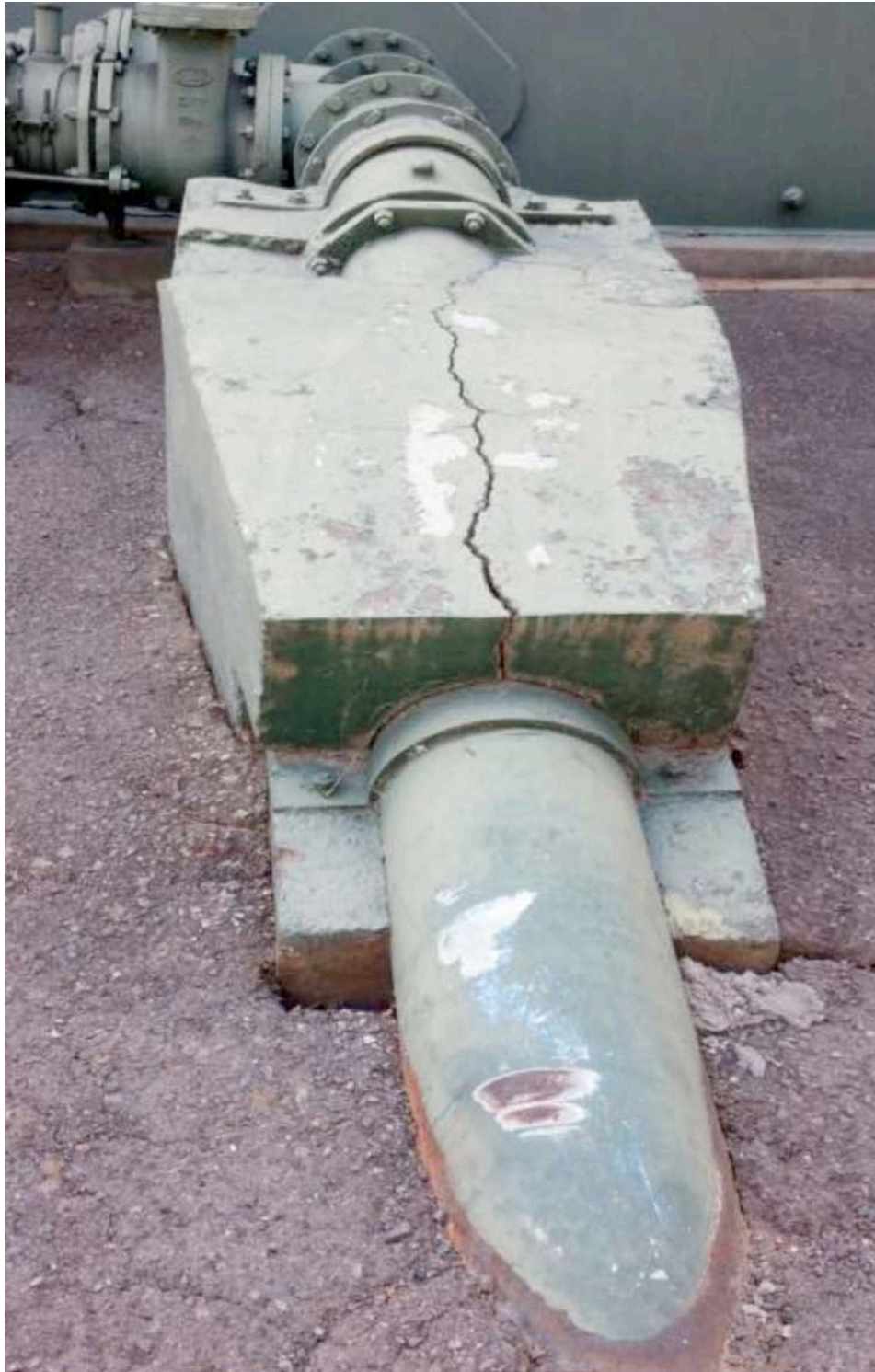
Figure B-28. Tank B. Inlet Outlet Pipes, Cracked Concrete Thrust Block
