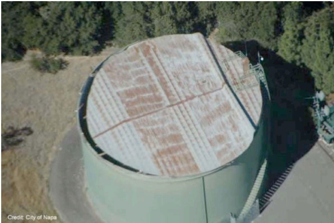
Figure B-25. Tank B. Damaged Corrugated Metal Roof
