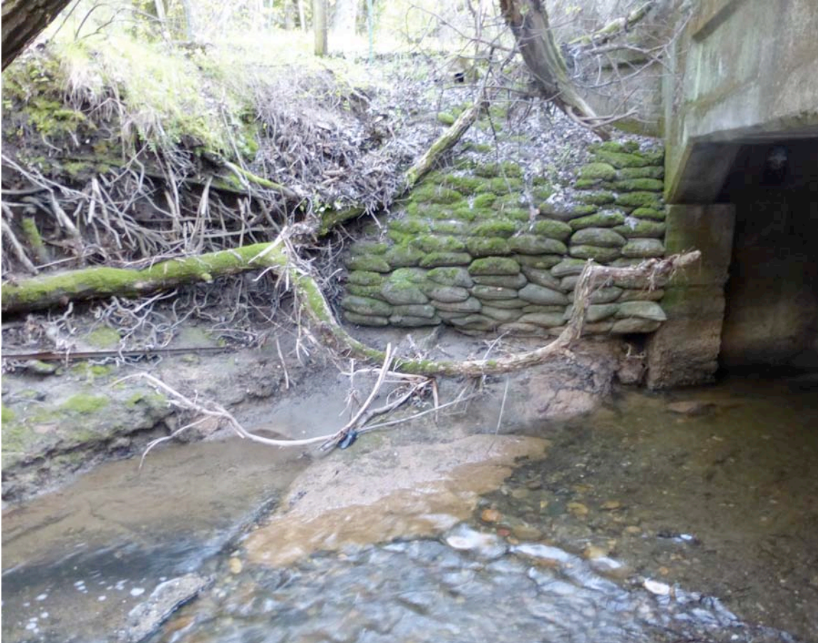
Figure 5-13. Matadero Creek crossing at Sta 33+43. View looking northerly. Slope rip rap is in place. Top of concrete-encased pipe is in foreground.
