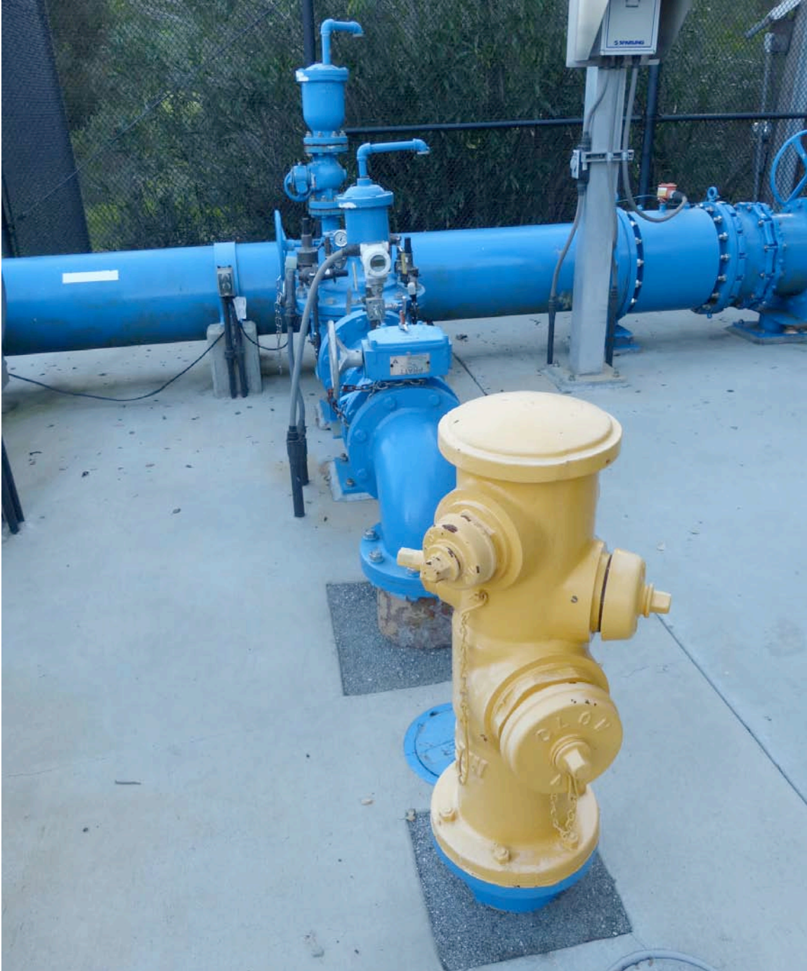
Figure 5-16. Pipes at Quarry Booster Pump Station. Asphalt-filled cut-outs in concrete pads.
