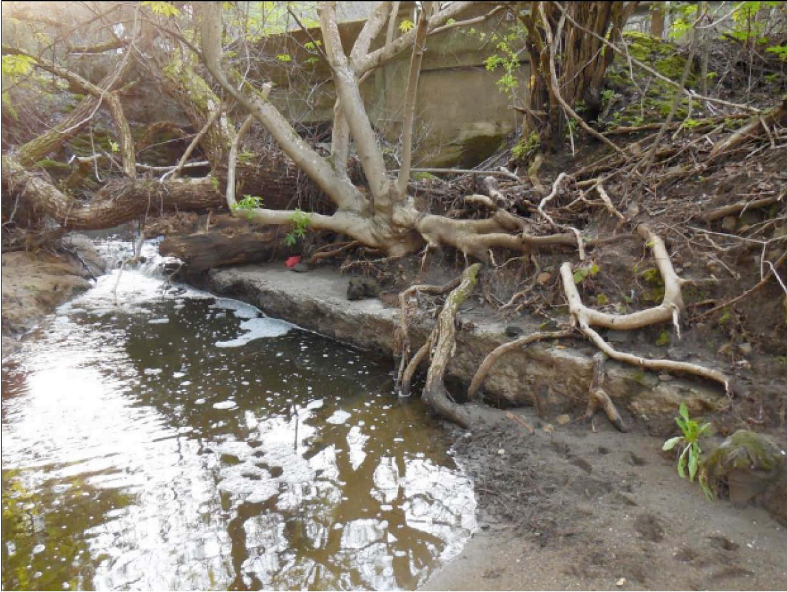
Figure 5-12. Matadero Creek crossing at Sta 33+43. View looking upstream (looking south). The exposed concrete encasement for the CCP is evident.
