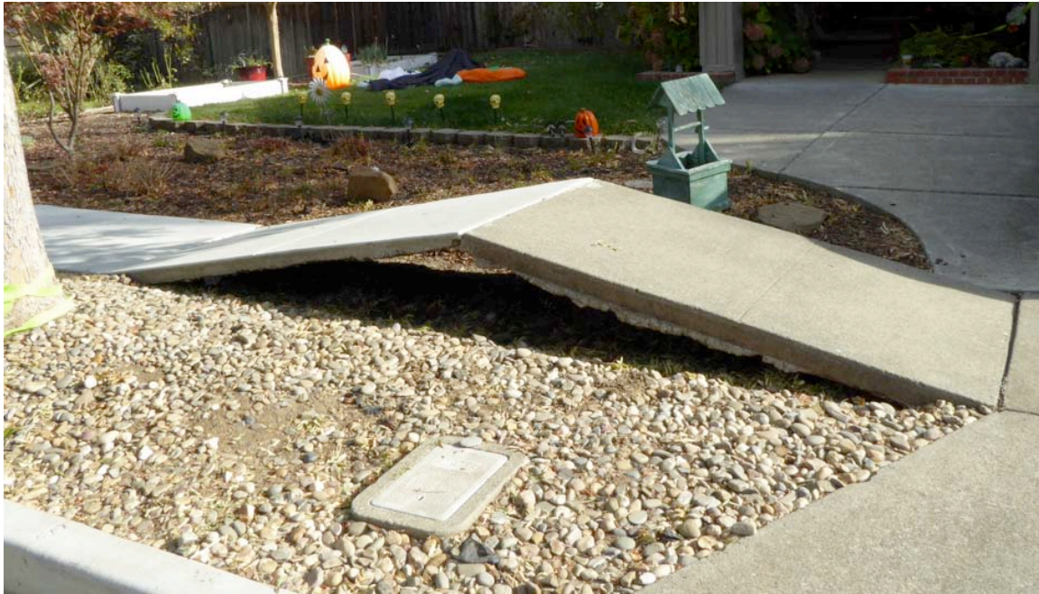
Figure B-9. Buckled Sidewalk at Fault Offset Location
