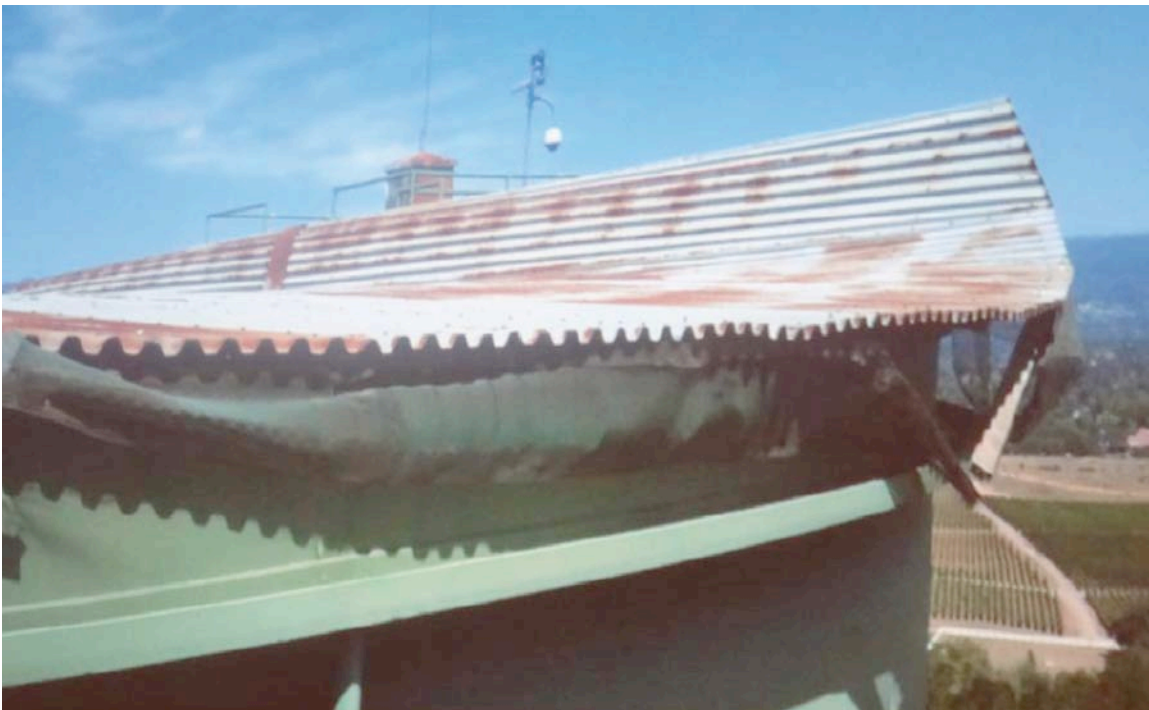
Figure B-26. Tank B. Corrugated Metal Roof Damage (Side View)
