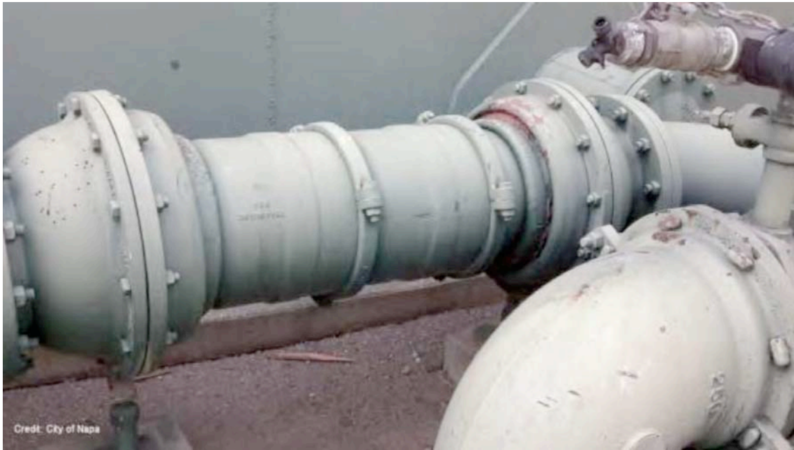
Figure B-27. Tank B. Inlet Outlet Pipes, Pipe with Ball and Slip Joints
