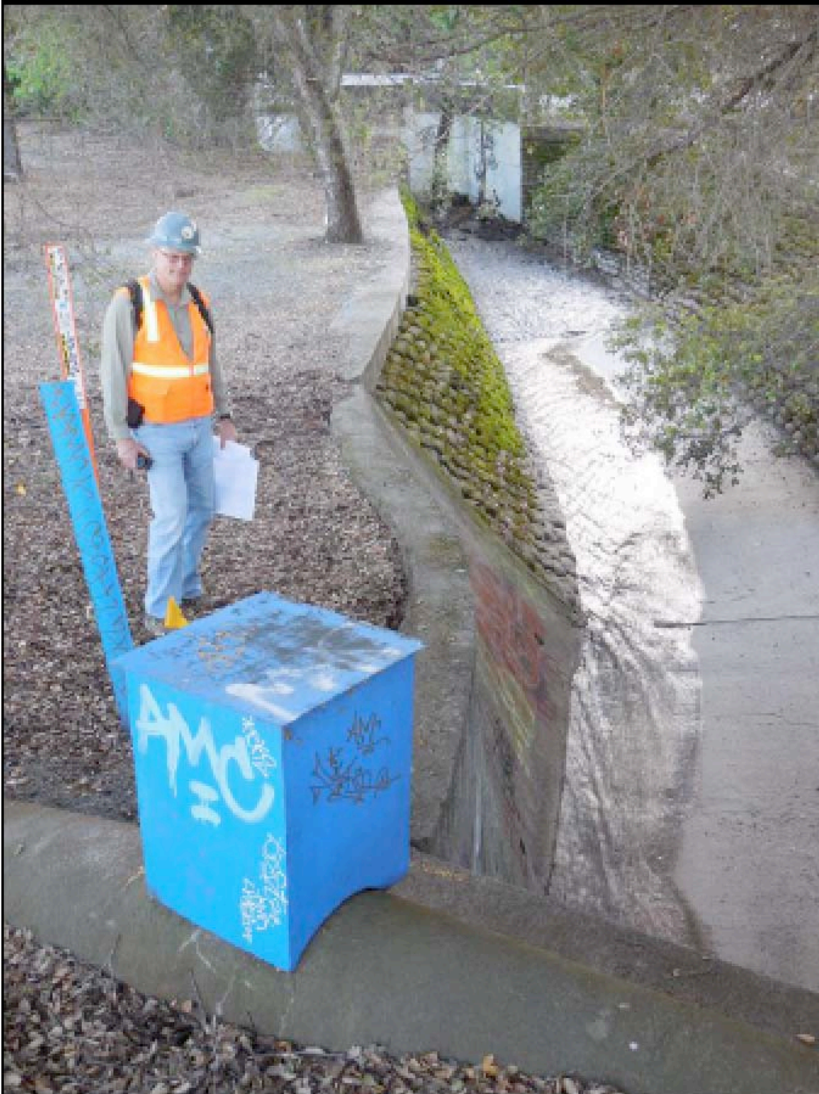
Figure 5-14. Matadero Creek adjacent to Quarry Booster Pump Station. View looking upstream (looking south). Pipe in foreground is inlet water pipe to Quarry booster pump station. Eidinger stands behind box presumed to house an air release valve.
