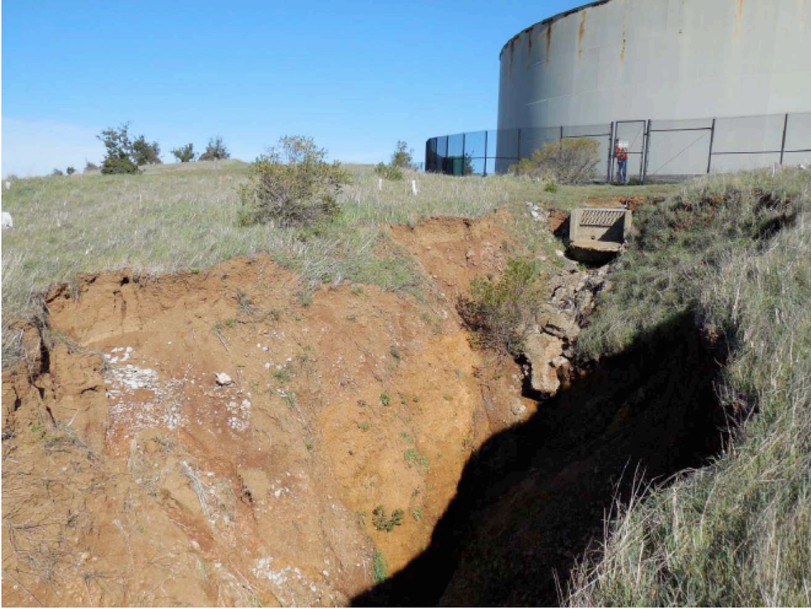
Figure 5-4. Active erosion and gully formed by storm drain, southeast side of reservoir
