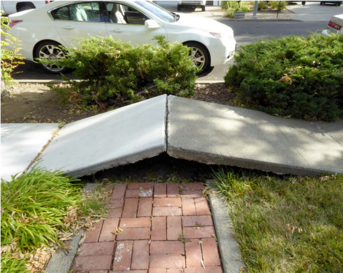
Figure B-10. Buckled Sidewalk at Fault Offset Location
