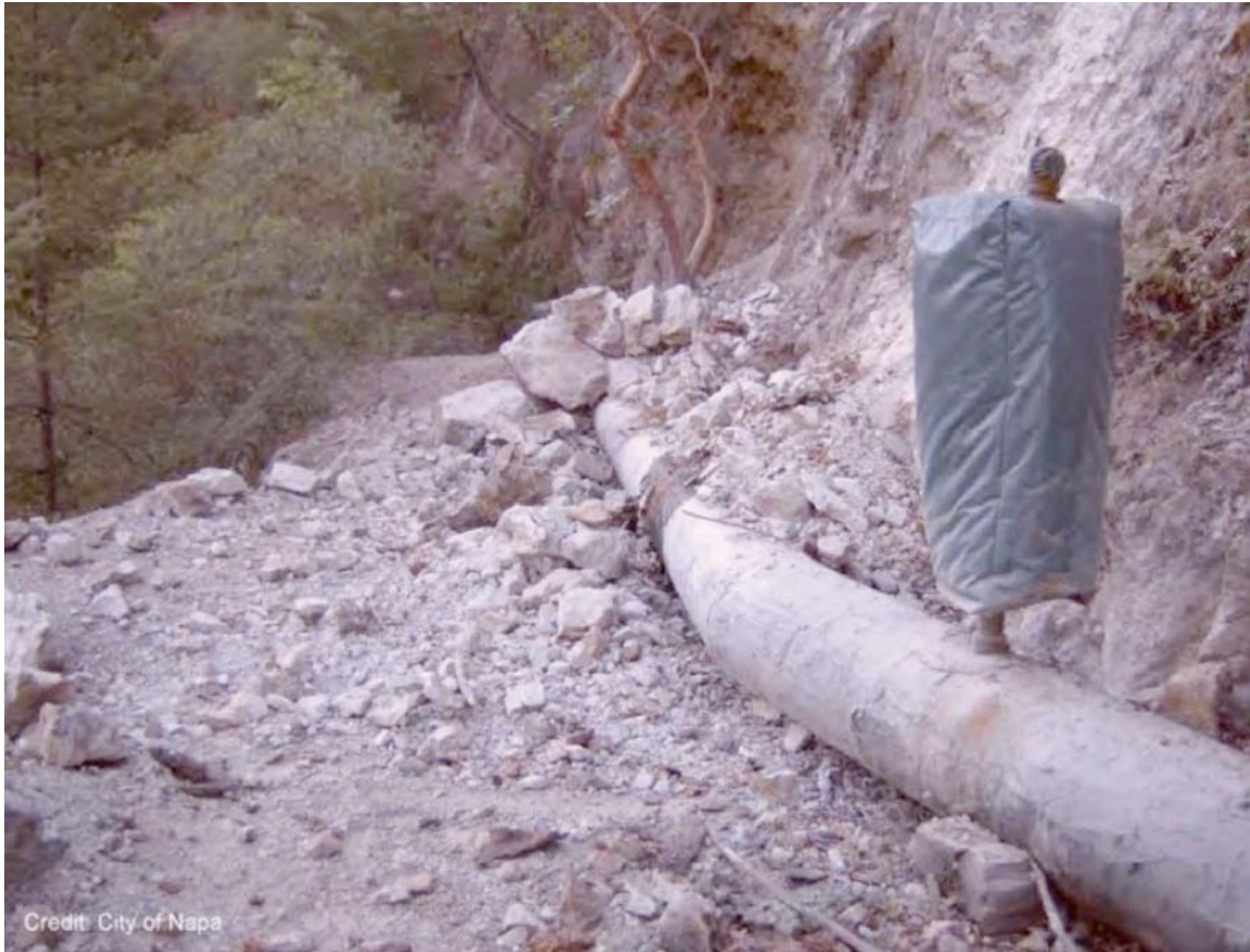
Figure B-24. Milliken Pipeline with Rockfall
