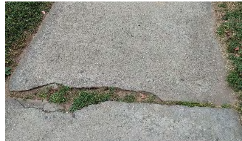
Exhibit 15: Sidewalk with Cracked Pavement and Vegetation
