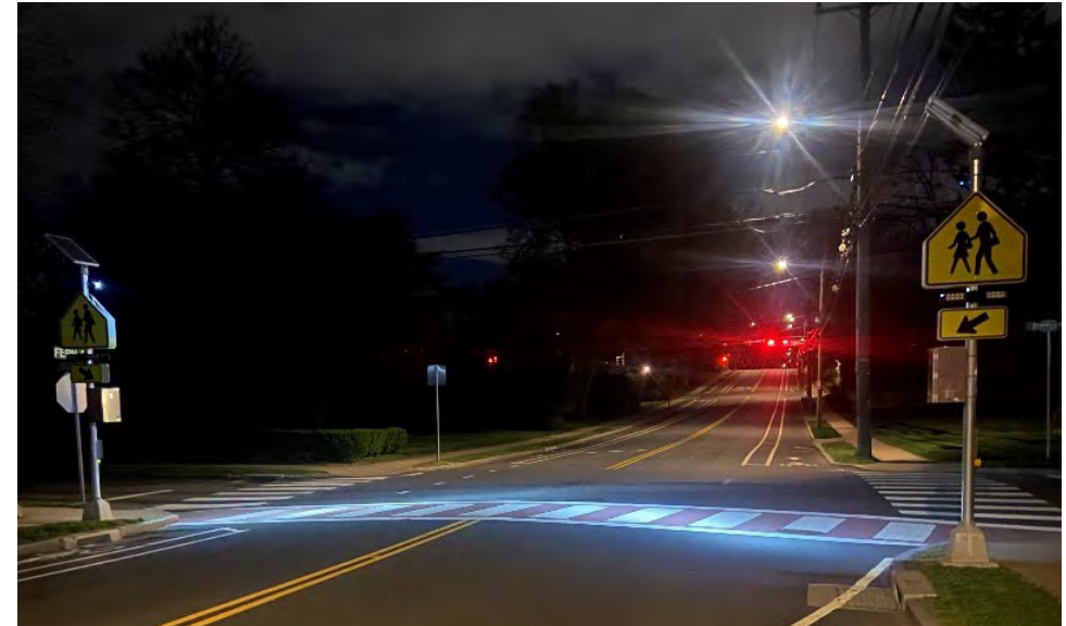
Exhibit 19: High Intensity Light with RRFB at Fern Street Crosswalk (Source: Town of West Hartford)
