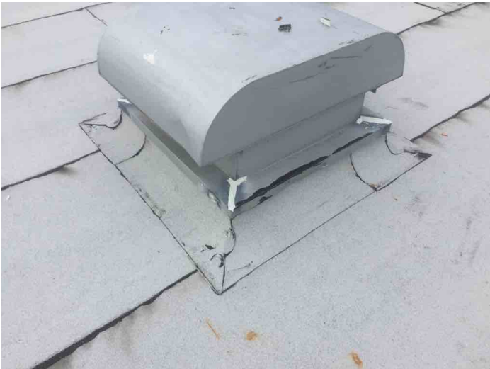
Group: 2.6 Category: Typical Detail Comments: Curb flashing
