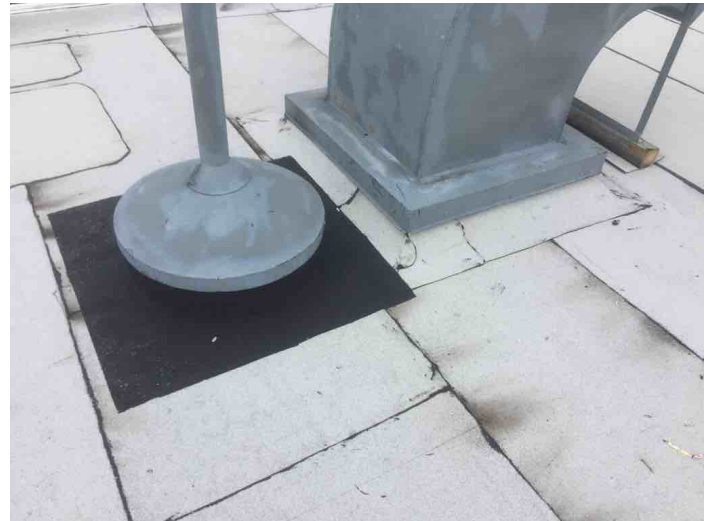
Group: 2.7 Category: Typical Detail Comments: PermaFlash application and curb flashing
