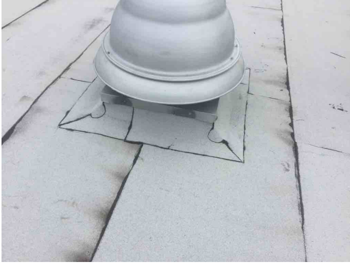
Group: 2.8 Category: Typical Detail Comments: Curb flashing
