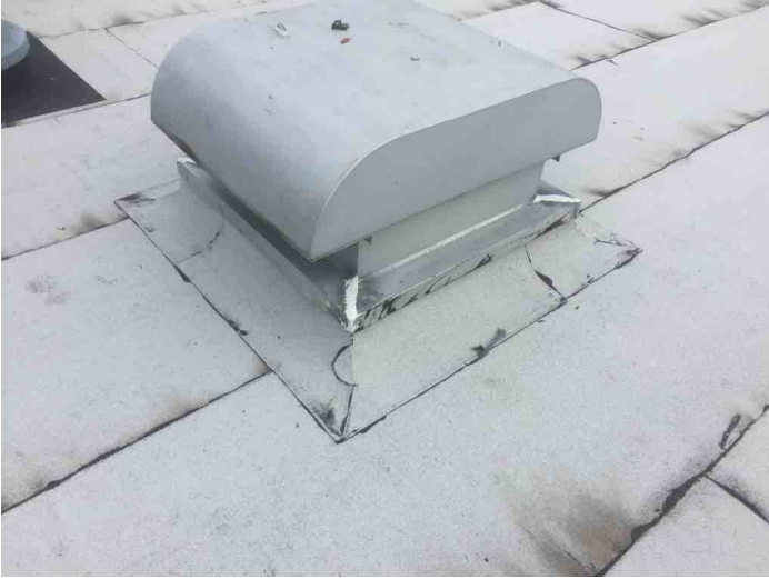
Group: 2.4 Category: Typical Detail Comments: Curb flashing
