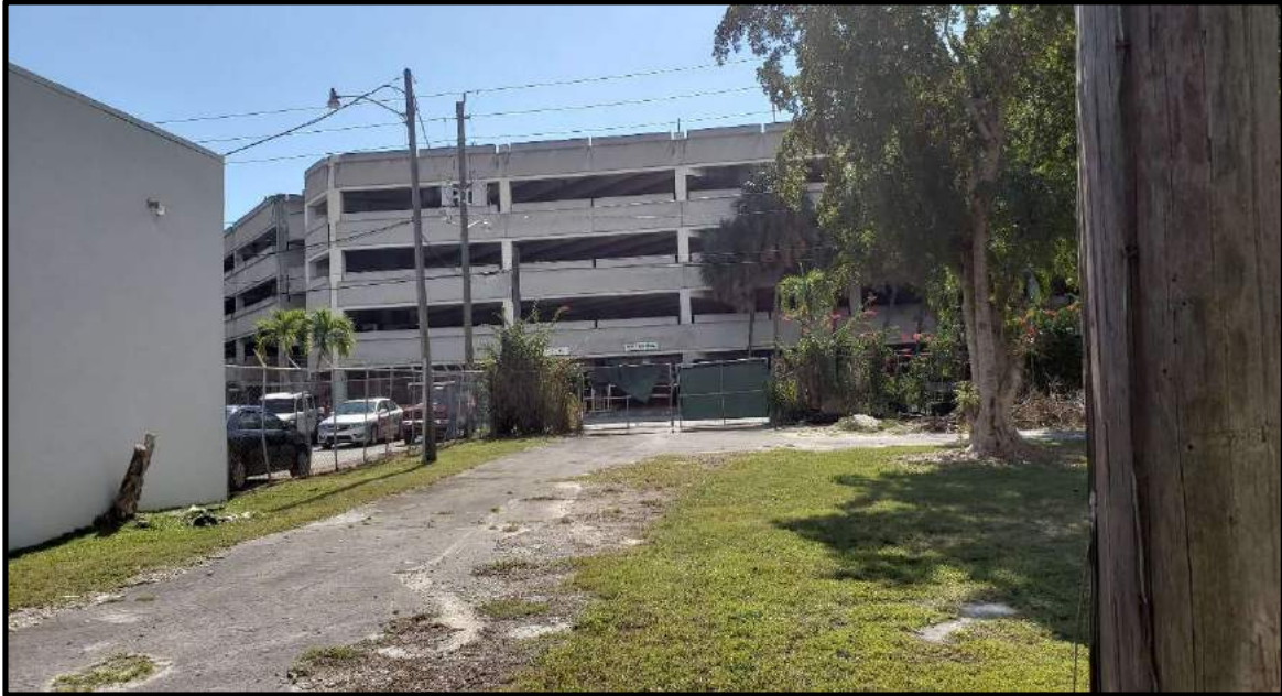
Looking South across the subject property at the South Miami Metrorail Parking Garage across SW 70 th Street.
