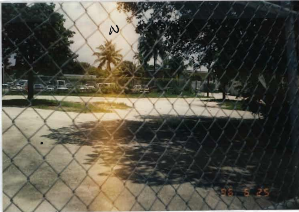
LOOKING NORTH - BUILDING (N2) AND YARD CLEARED AND CLEANED OF ALL WASTE, MACHINERY & EQUIPMENT
